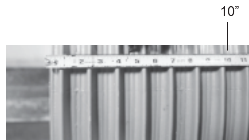
Measure & mark the location for the center of the discharge hole. Location shown is for Anchorage Tank steel liftstation tanks.
