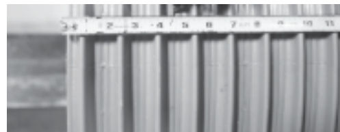
Measure & mark the location for the center of the discharge hole.
