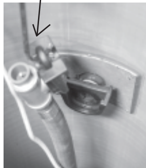
Make a smooth, continuous fillet around the seam between the mounting plate and riser.
