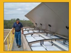
The AX-Mobile uses textile sheets in a packed bed media filter. It can treat blackwater and greywater to a level where effluent can be reused for surface or subsurface irrigation or for dust control (as regulations permit).
