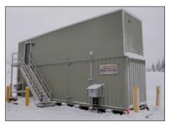
had to meet strict NPDES permit requirements for surface discharge, since subsurface discharge was not an option. The system was commissioned in December 2009 and sampling shows that effluent quality is averaging BOD of 6 mg/L, TSS of 5 mg/L, and fecal coliform of 5.9 MPN/100 m/L.
