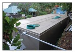
12,000 pounds (5443 kg), the units were trucked to the site, down steep narrow roads, on the back of a standard flatbed and lifted with a crane. Less than two days after reaching the site, the system was up and running, in spite of power fluctuations and other problems. This system includes a UV disinfection unit, and effluent sampling shows it is producing 7 mg/L BOD. An addition to the treatment systems is currently in process.
