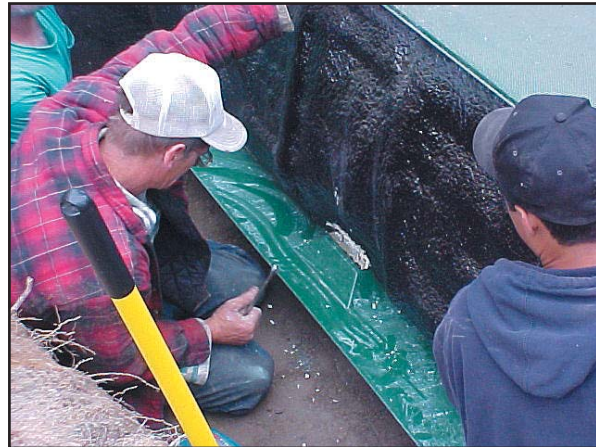
Tilting the Filter on one side to bolt on the flange.
