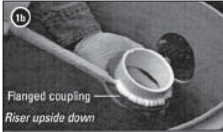
Applying adhesive to the coupling.
