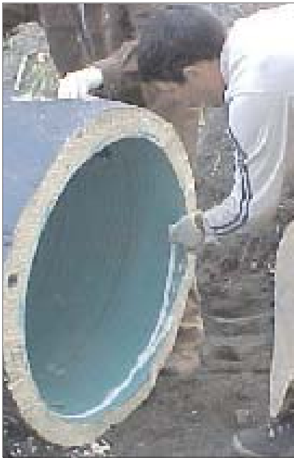
Apply adhesive to the outer edge of the adapter
