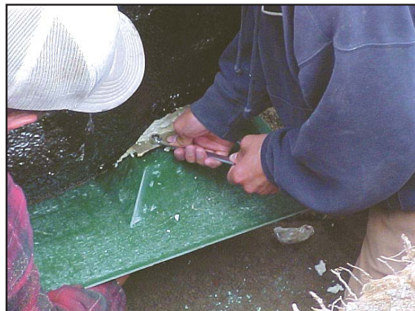
Tilting the Filter on one side to bolt on the flange.
