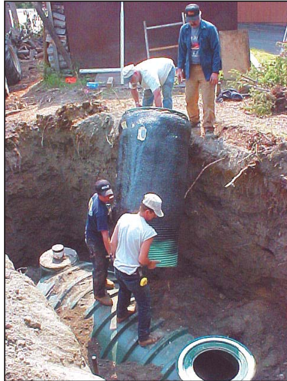
Moving the riser into position
