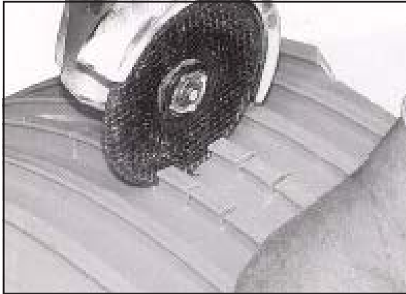
Grinding access riser ribs
