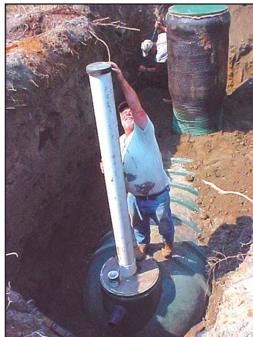
Installing the clean-out
