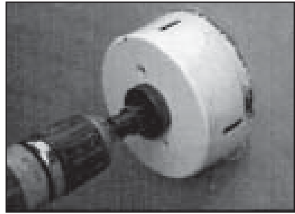
Drilling hole for the RSV
