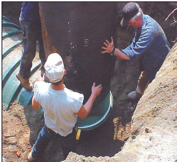
Spin the riser to face the desired direction
